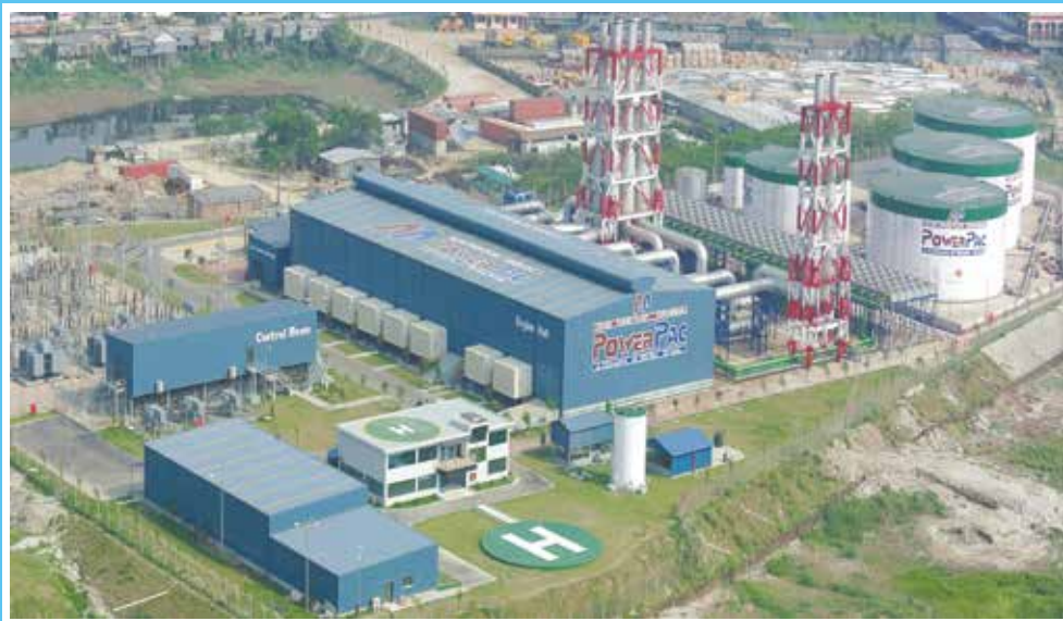
A view of the 100 MW HFO Fired Keraniganj Power plant
